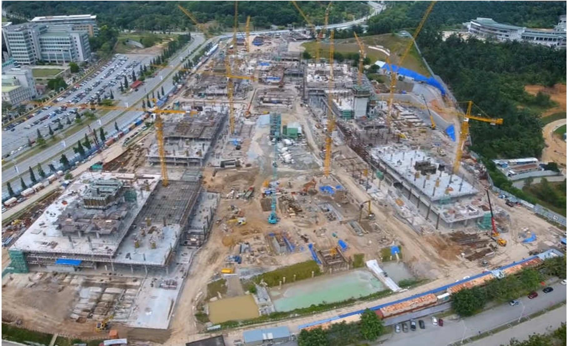
Parcel F , Putrajaya : aerial view of present progress
